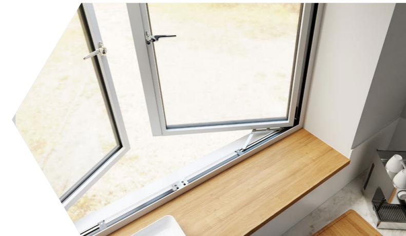
The ultra slim 59mm sightlines of the innovative Classic window system maximises the light flooding into your home, creating a refined architectural look. While our patented construction method – using threaded screws to bind corners tightly together in perfect unison – creates perfect run through mitres on internal joints, doing away
